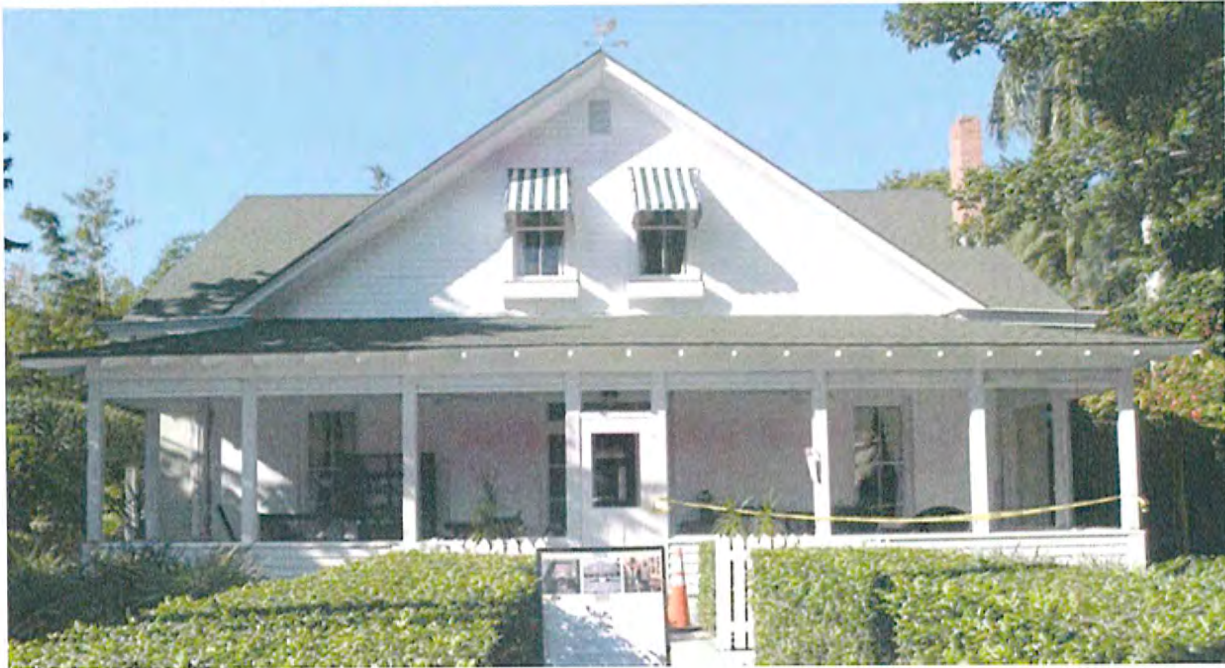
Photo D: Front-facing gable roof
