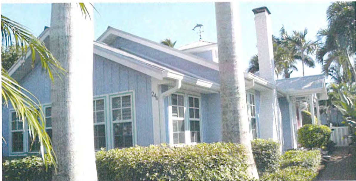
Photo T: Vertical board and batten siding
