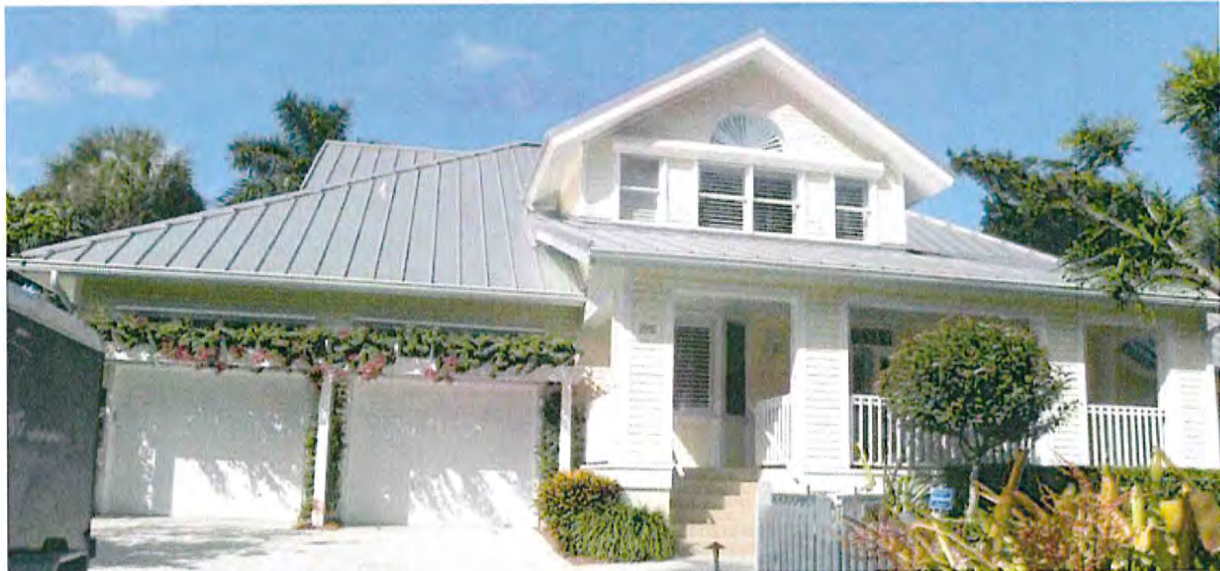
GABLE: 99 11 th Avenue South
