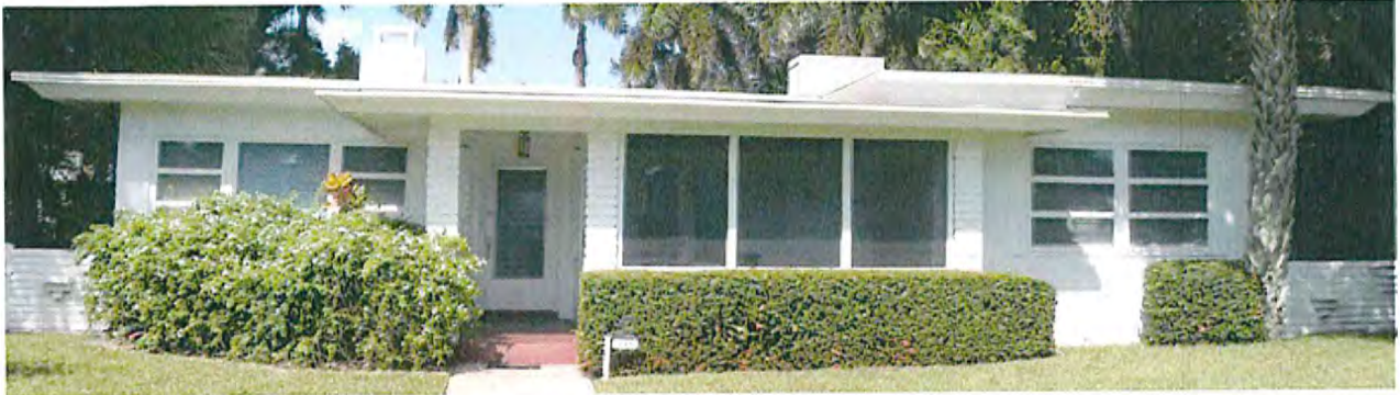
SHED: 241 10 th Avenue South
