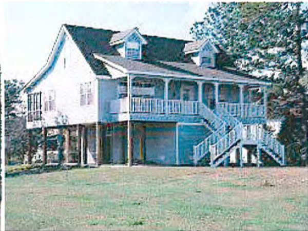
Photo R: Pier foundations (main floor elevated above the ground)
